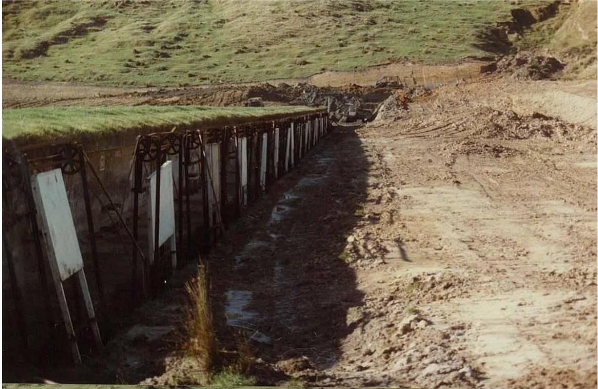
Seddon Range, 1984. The old Hythe pattern frames await removal as the area is prepared for new target hoists. Note the hillside partially removed to accommodate the extended range. (NRANZ)
